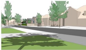
CONTEXT VIEW ALONG MALLORY ROAD LOOKING SOUTH
