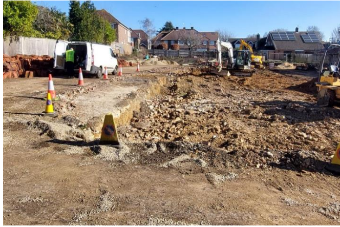
Northern part of the site
