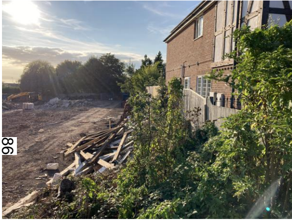
North boundary of the site with No.6 Mallory Road
