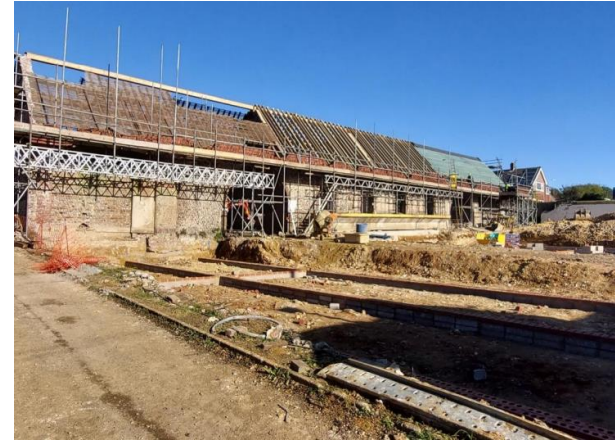
Southern part of the site fronting The Droveway
